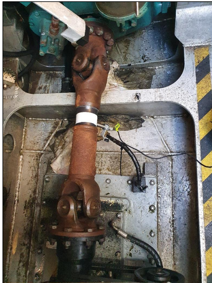
Figure 66: W4W: Waterjet Installation Situation
